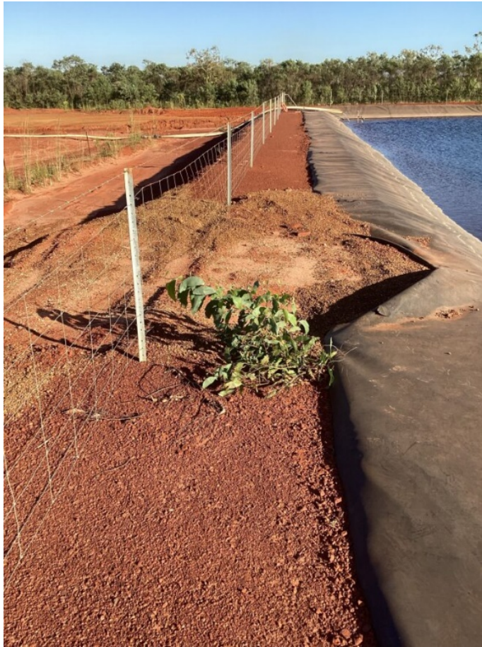
Figure 16: Process Water HDPE Liner Requiring Repairs
