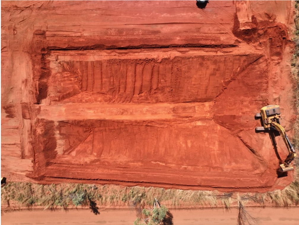
Figure 2: Landfill Cell Construction
