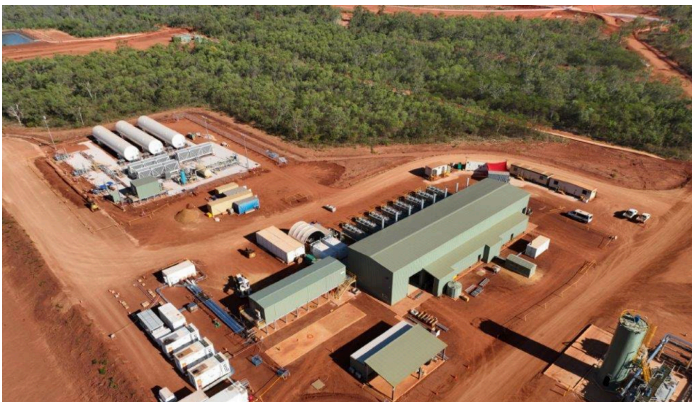
Overview of power station and LNG storage infrastructure
