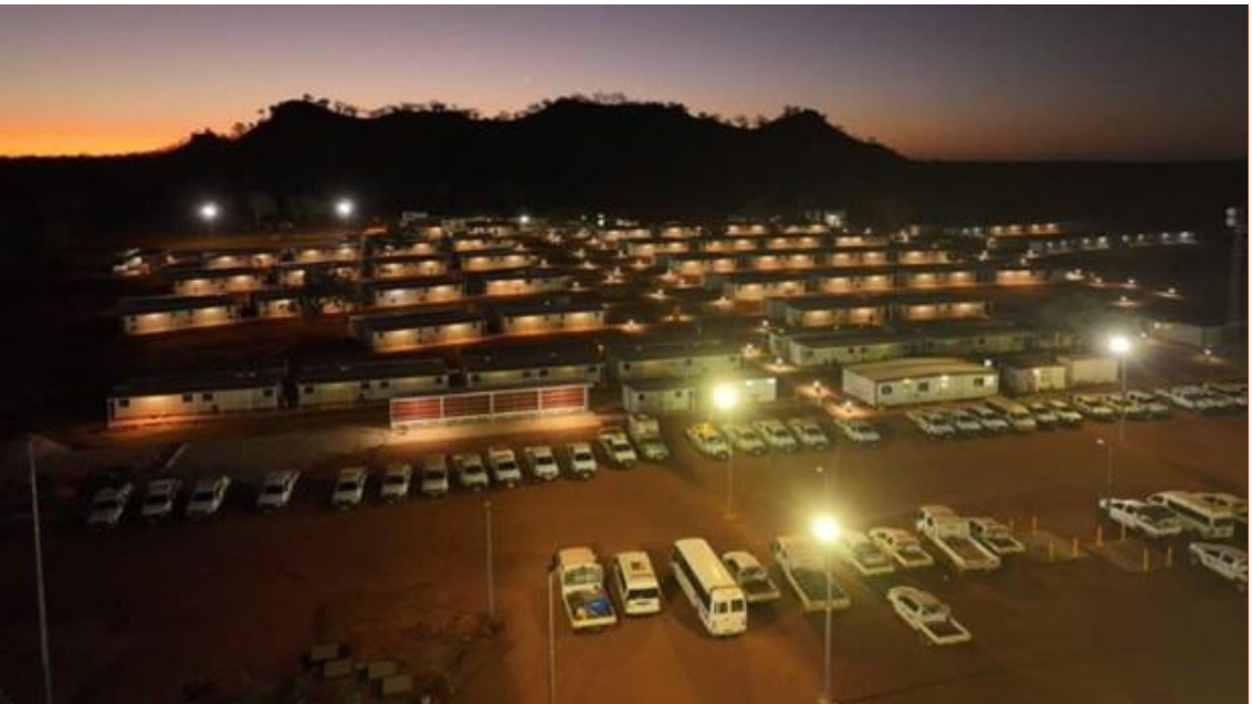
The Thunderbird Accommodation Village was completed and handed over the KMS.
