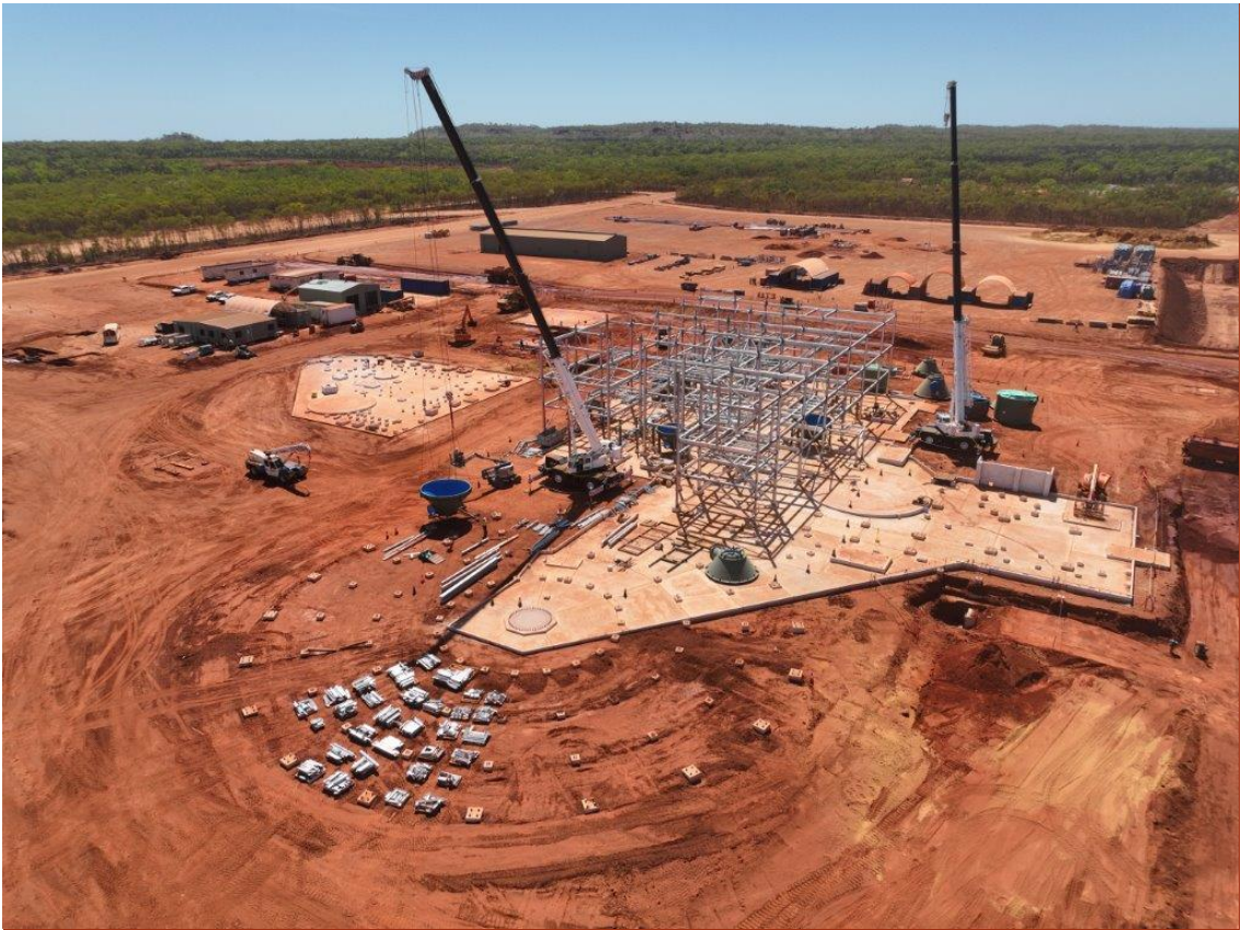
Construction activities at the Thunderbird Mineral Sands Project
